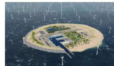
The Power-to-X Island will have ca. 200 turbines attached to its grid, producing 3-gigawatt power (equivalent of 3 million households in Europe). Is it the right way to go; only time will tell!
