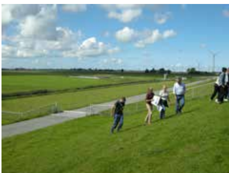
From the seadike view on the double dike
